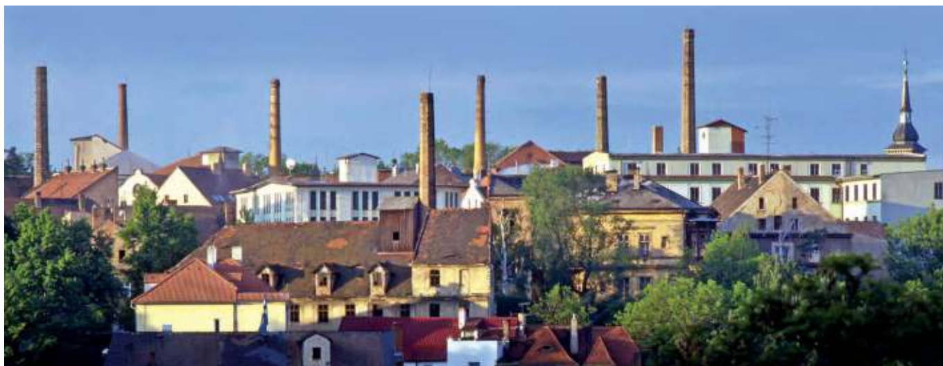
Žatec, view of the characteristic panorama of the Prague Suburb with hop processing buildings and their chimneys, “forest of chimneys”. Photo by V. Mach
