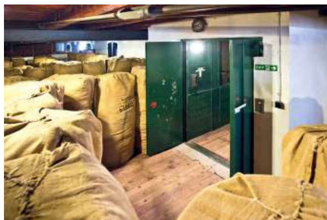
Žatec, Prague Suburb – additionally installed typical electric freight elevator for transporting hop bales, house No. 305 on Prokop Velký square. Photo by V. Mach
