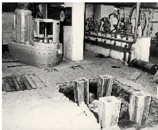
Installation of the TMS pelletizer Instalace granulátoru TMS
